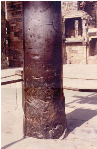
Iron Pillar at Delhi. Fig. 3 Hammer marked cavities are still visible on the surface of the pillar in the rough region. The rough region was originally buried under the ground when the pillar was located at Udayagiri.
